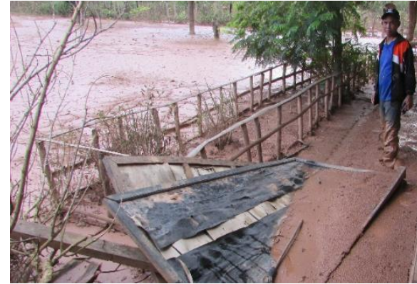
Damaged school building and equipment at Sanamxay, Attapeu. Photo credit: Save the Children International staff
