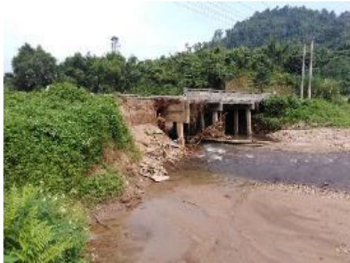
Bridge on R3 (Photo on 6 October 2018)
